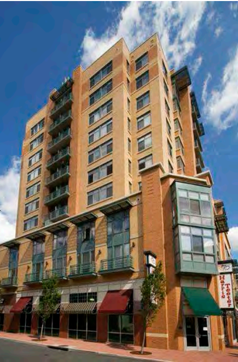
The Delancey Apartments – Arlington, VA 525 sliding window, 750 fixed window 900 casement window, 1400 terrace door 1420 dual terrace door Comfort E2, custom color insulated panels Dwarf Spruce custom powder coat finish
