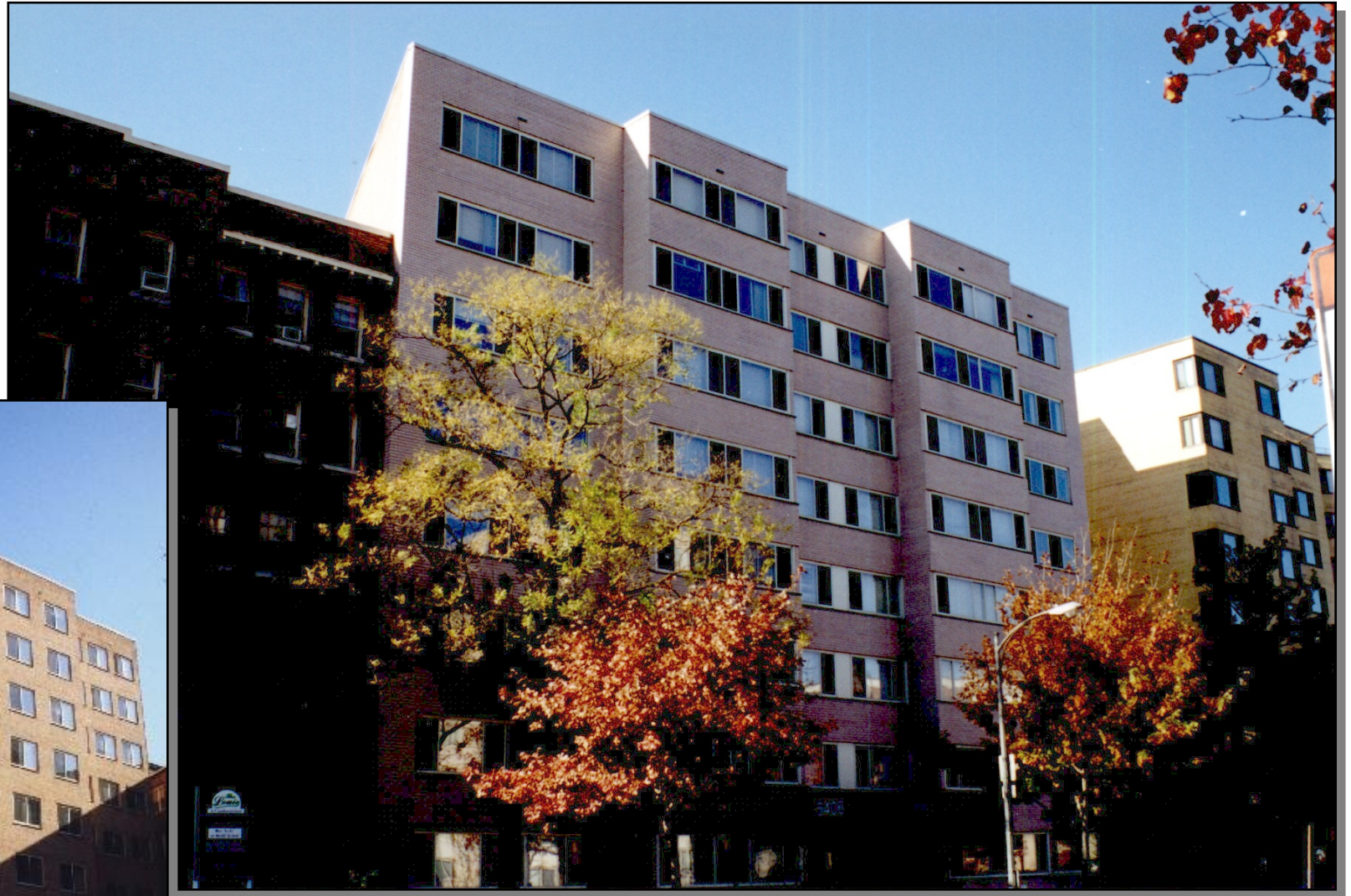
Chase Plaza, Washington, DC – 8 floors Series 525 and 530 Horizontal Rolling Creme powder coat finish
