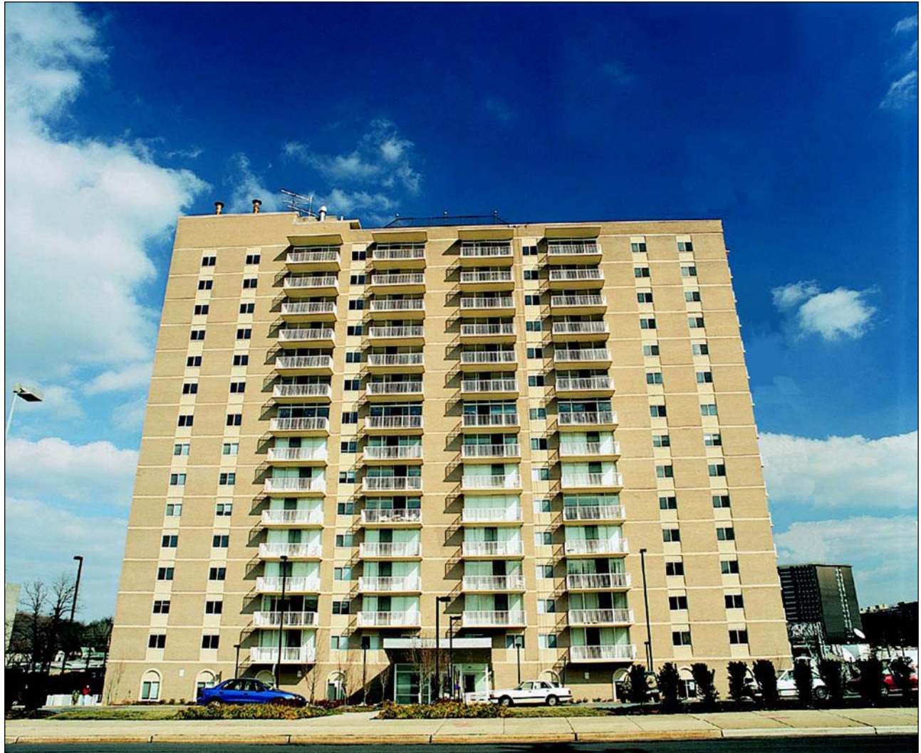
Westwood Towers, Bethesda, MD – 15 floors Series 525 Horizontal Rolling; Series M-2000 Sliding Glass Doors Clear Anodized finish
