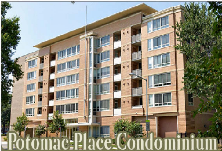
Potomac Place Condominium Oxon Hill, MD Collingwood Custom Powder Coat Finish
